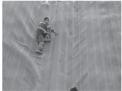
Photo 2. Geocomposite drainage fixation on the slope.
