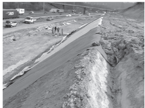
Photo 3. Mechanical fastening at the summit with anchoring.
