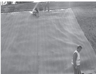
Photo 1. Geocomposite drainage unrolling.
