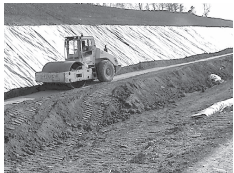
Photo 4. Filling and under-steeping the slope.
