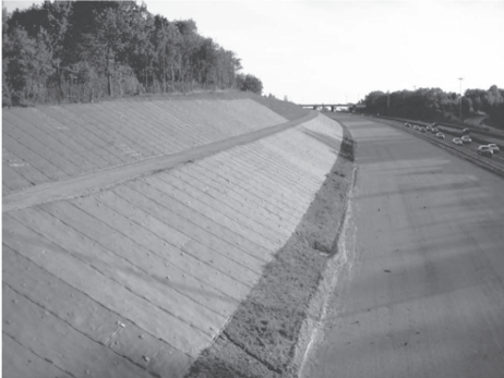
Photo 5. Filling and under-steeping the slope.
