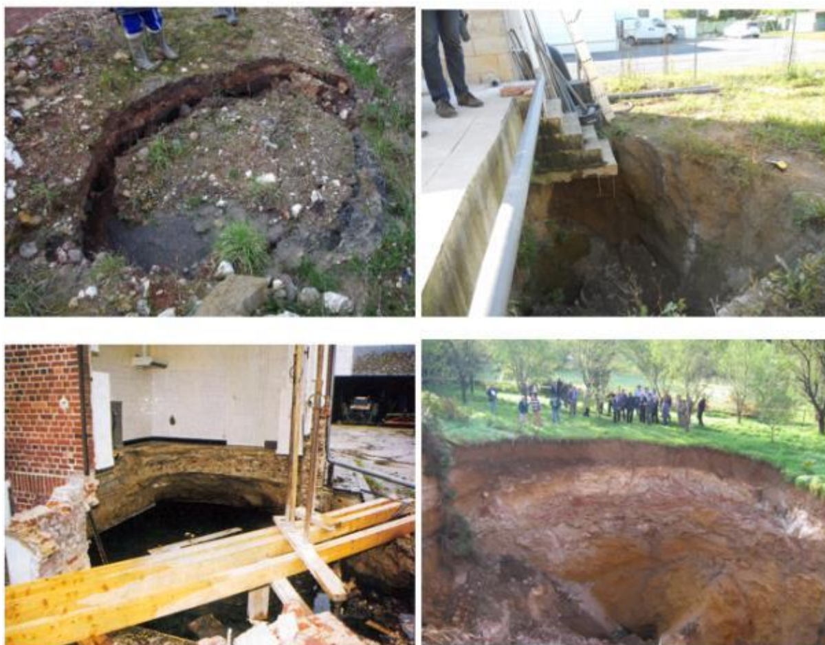
Figure 9 : Examples of local collapses near man-made cavities - source: Ineris
