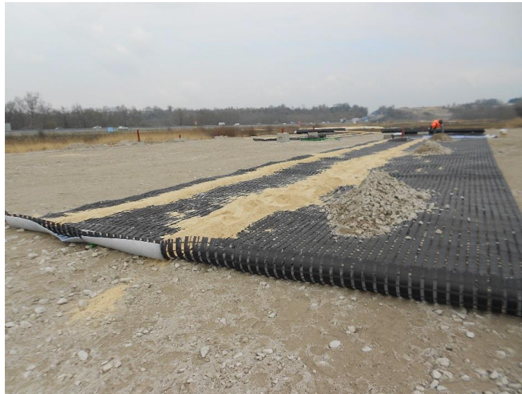
Figure 34 : Example of an instrumented geosynthetic installation - Source: Afitexinov
