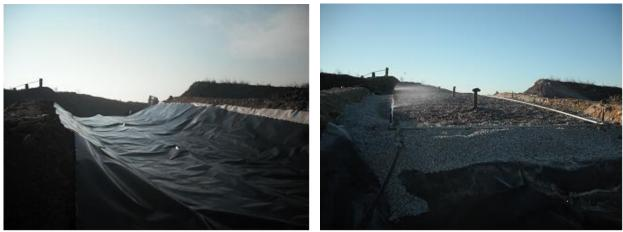
Figure 5: Geomembrane installation
