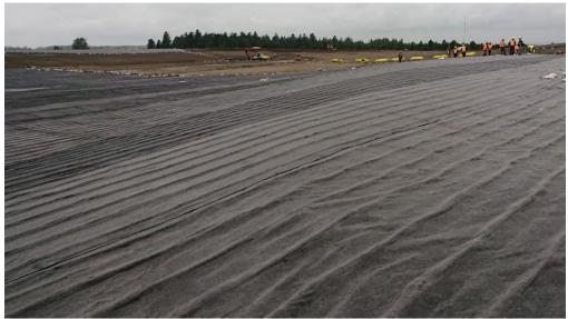
Figure 2. Drain Tube installation
