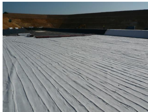
Figure 2 Leachate drainage at the bottom of landfill
