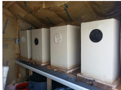
Figure 10 Constructed flow boxes
