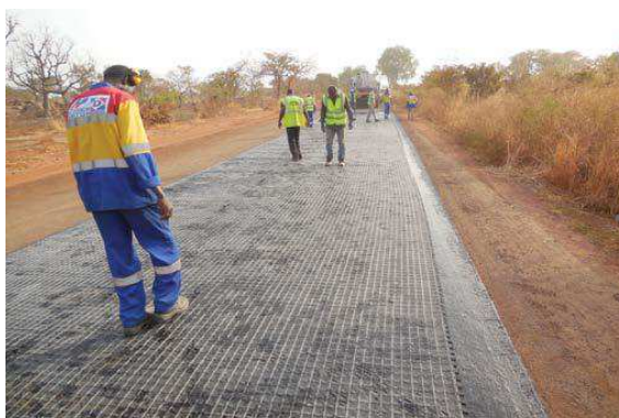
Figure 7: Laying of a coated geosynthetic combining fiberglass geogrid and light veil (GG/veil C 100x100) on RN1 in Burkina Faso in 2015.
