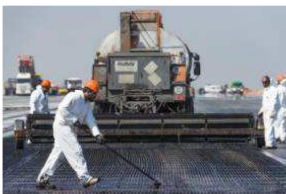
Figure 8: Laying of the coated geosynthetic combining fiberglass geogrid and light veil (GG/veil C 100x100) on runway 2 of Paris CDG airport in 2016. Picture courtesy of Colas.
