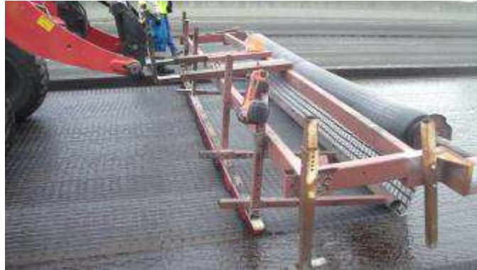
Figure 9: Laying of the coated geosynthetic combining fiberGlass geoGrid and light veil (GG/veil C 100x100) on French highway A7 in 2017.
