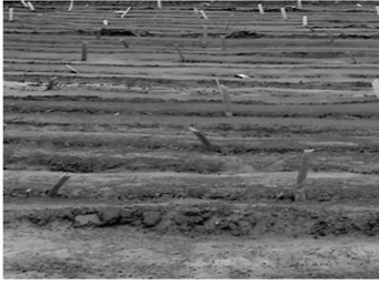
Photo 1. Installation of the geosynthetic vertical drains.
