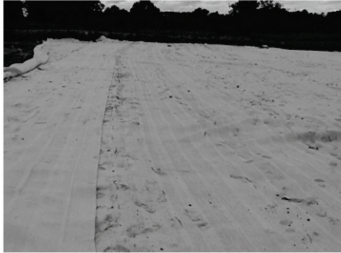
Photo 2. Horizontal geocomposite drainage.
