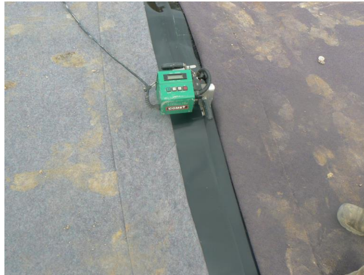
Figure 10: Longitudinal welding of Protecterre PF between two rolls.
