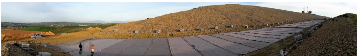
Figure 7: Installation of waterproofing geocomposite on railway platform near Larache (Sector 3)
