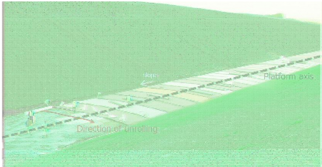
Figure 8: Direction of installation depending on the slope of the platform
