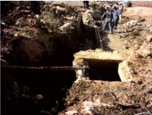
Figure 7. View of the various utility networks
