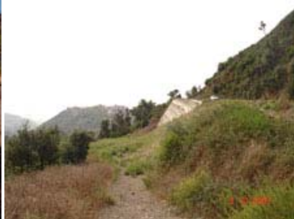
b. Construction when completed
