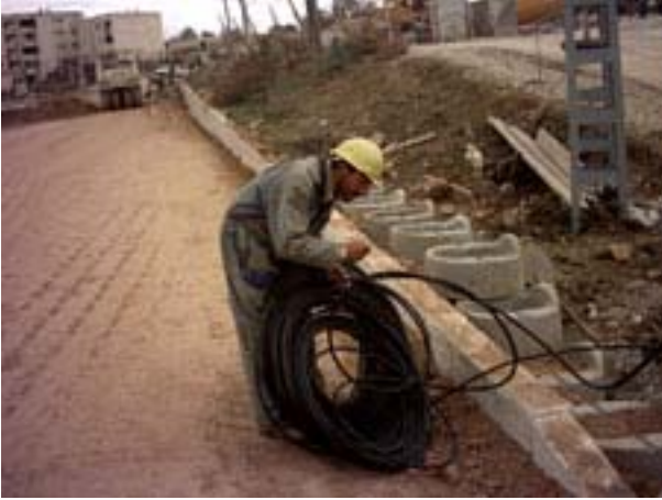
Figure 11. Installation of the watering system
