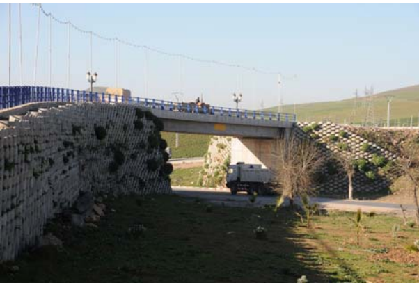
Figure 12. The completed construction
