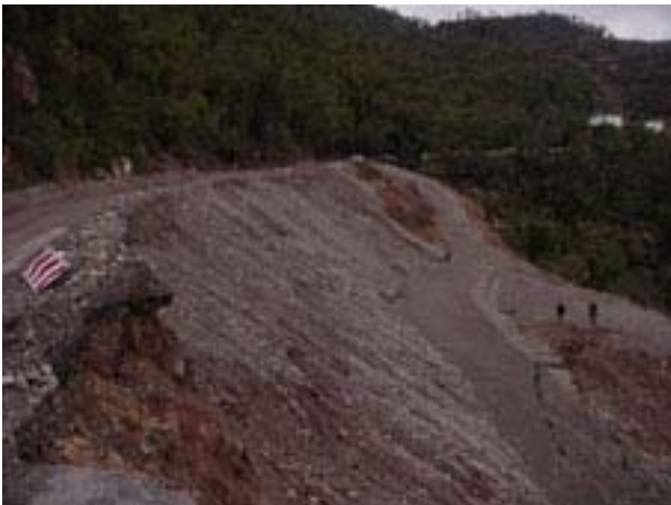
Figure 3. Longitudinal cracks which appeared due to the load of new soil
