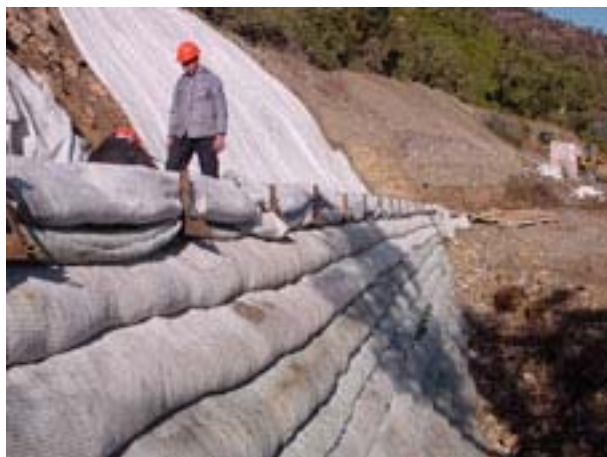
a. Construction in progress
