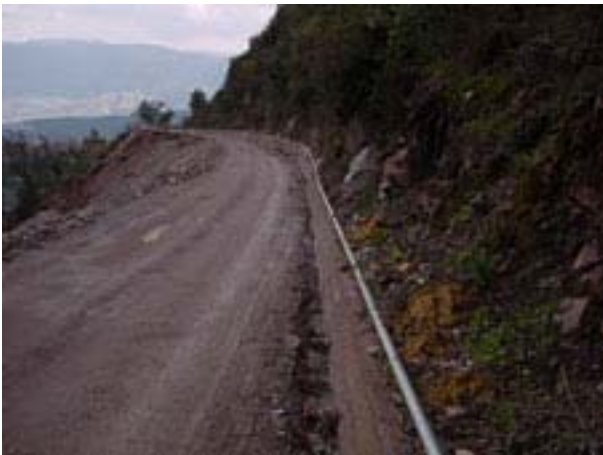
Figure 1. View of the landslide
