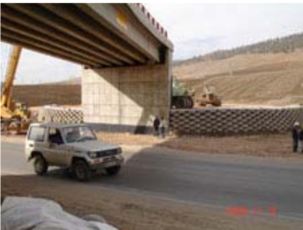
Figure 10. View of the work in progress
