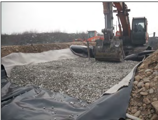
Figure 17. Construction of test site
