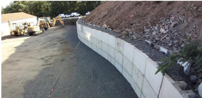
Figure 4. Test working site.
