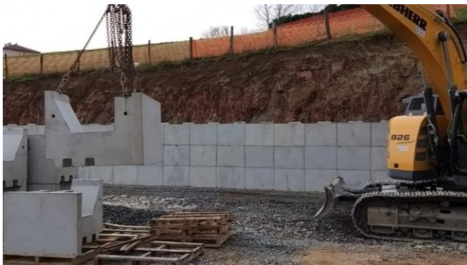
Figure 2. Illustration of the block-lifting process.
