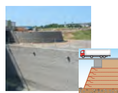
Retaining walls, road and rail bridge abutments
