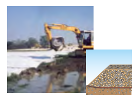
Embankment on low bearing capacity soils
