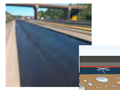
Rehabilitation of damaged pavement, cracks control/mitigation
