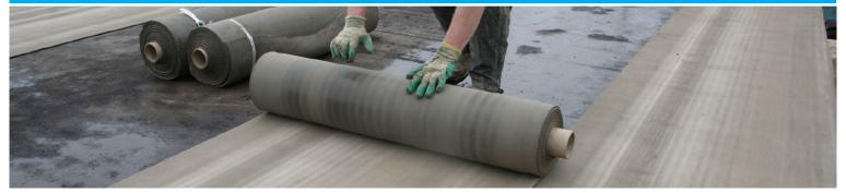
Concrete Canvas® is part of a revolutionary new class of construction materials called Geosynthetic Cementitious Composite Mats (GCCMs). It is a flexible, concrete filled geosynthetic that hardens on hydration to form a thin, durable and waterproof concrete layer. Essentially, it's concrete on a roll™. Concrete Canvas® GCCM (CC) allows concrete construction without the need for plant or mixing equipment: just add water.
