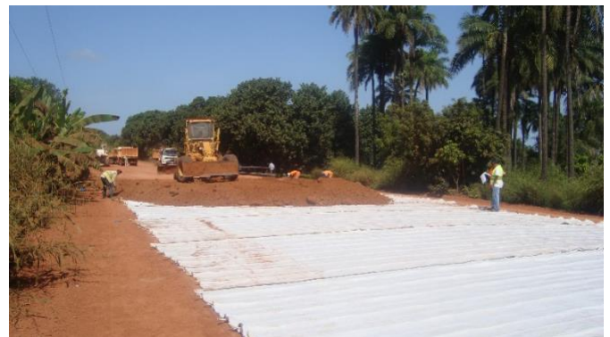
Backfilling in the overlapping direction
