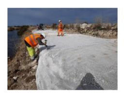
Preparation on substrate, cutting and stitching of geogrids
