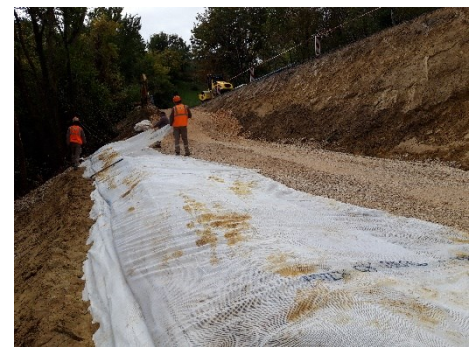
Backfill on the geogrid, installation of the return and manual pre-tensioning
