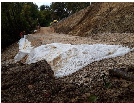
Backfill on the geogrid, installation of the return and manual pre-tensioning
