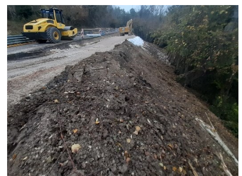
Backfill on the geogrid, installation of the return and manual pre-tensioning
