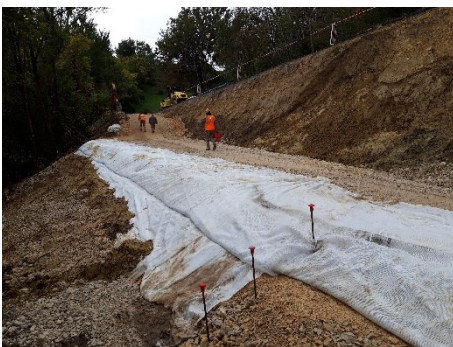
Backfill on the geogrid, installation of the return and manual pre-tensioning
