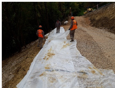
Backfill on the geogrid, installation of the return and manual pre-tensioning
