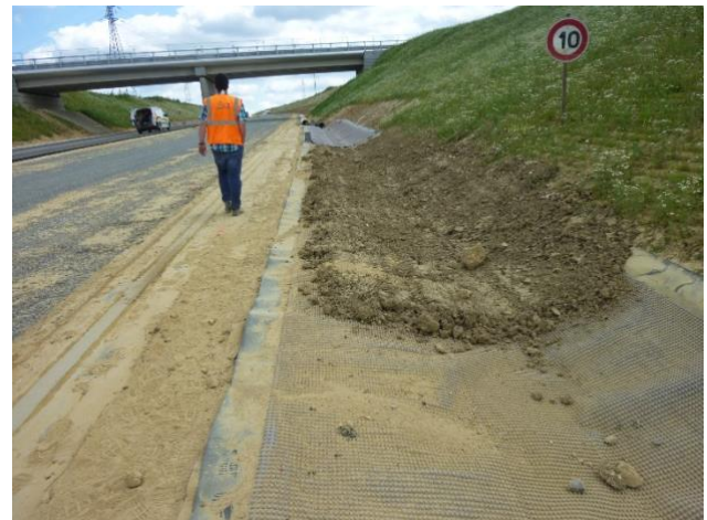
Stabiliner Alveo backfilling (overlapping installation)
