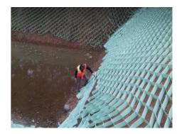
Adjustment and installation of anchor pegs according to design calculations
